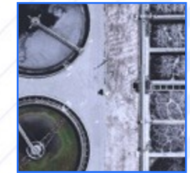
Water and Wastewater Systems
